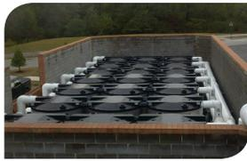
*An ice storage system reduces energy costs by shifting peak cooling loads to off-peak hours.*
