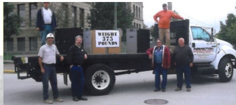
New 375 lb. courthouse boiler
