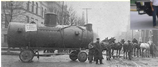
Original 22,000 lb. courthouse boiler
